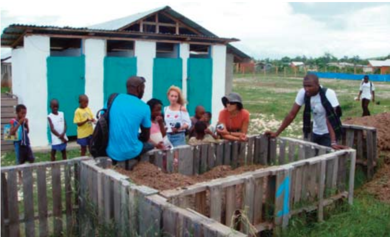
Figure 25: The toilets at the Matt Gunn orphanage site are located adjacent to the compost bins. There is no odor and no flies. A bagasse pile nearby provides the cover materials.
