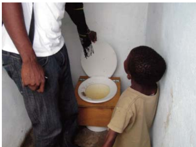
Figure 26 (above): The orphanage toilet is painted with a picture of the “human nutrient cycle” as well as a “GiveLove ecological sanitation” emblem. The rain water catchment system provides wash water for hands and toilet receptacles. GiveLove.org provided the setup and training for this self-managed compost sanitation system.
