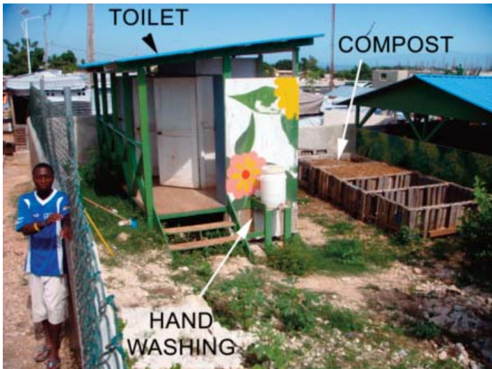
Figure 7 (above): A toilet stall at the Amurt school, located next to the compost bins.
