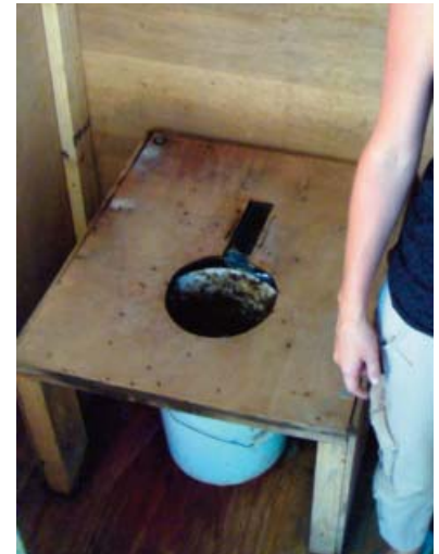
Figure 1: A "bucket toilet" uses no cover material, is very odorous, breeds flies and pollutes the environment. This feces-caked bucket in Port au Prince is an example of unacceptable sanitation.
