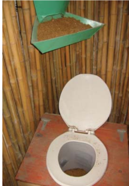
Figure 30 (right): Sopudep uses 20 liter receptacles that lift out of the toilet when full. The bagasse is dispensed by hand from the green wall-mounted bin.
