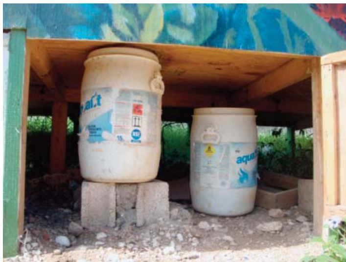
Figure 9 (above): 60 liter receptacles slide out from underneath the toilet stalls.
