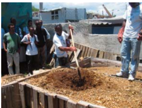
Figure 14: The compost pile is opened before fresh toilet material is added.
