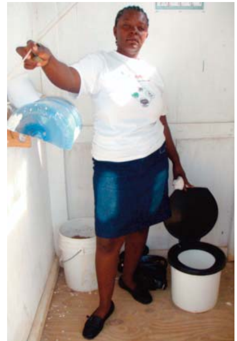
Figure 8 (right): This lady keeps the toilets clean at the Amurt School. The toilet material enters the below-floor receptacle through the white chute.
