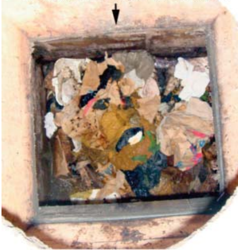
Figure 23: A typical Haitian pit latrine in Leogane at a Habitat for Humanity site is filthy and unpleasant. The toilet smells terrible, breeds maggots and flies, creates waste and pollutes ground water.
