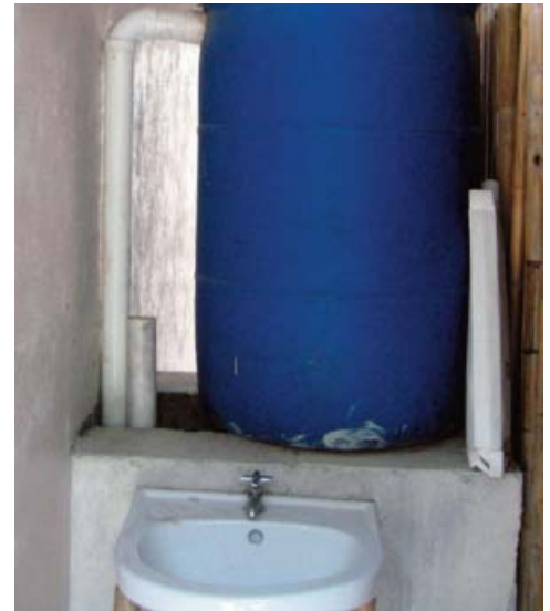
Figure 31 (above): Sopudep's toilet building includes a hand washing station supplied by rain water.
