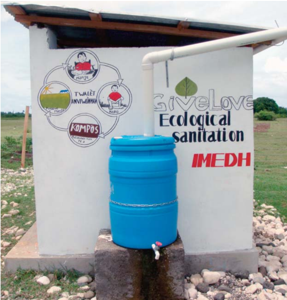
Figure 26 (above): The orphanage toilet is painted with a picture of the “human nutrient cycle” as well as a “GiveLove ecological sanitation” emblem. The rain water catchment system provides wash water for hands and toilet receptacles. GiveLove.org provided the setup and training for this self-managed compost sanitation system.
