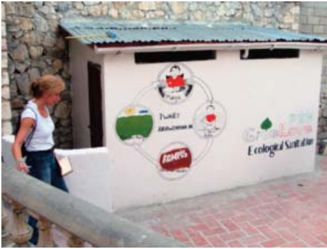
Figure 29 (above): The toilet system at the Sopudep School utilizes the same procedures as Amurt and Matt Gunn.
