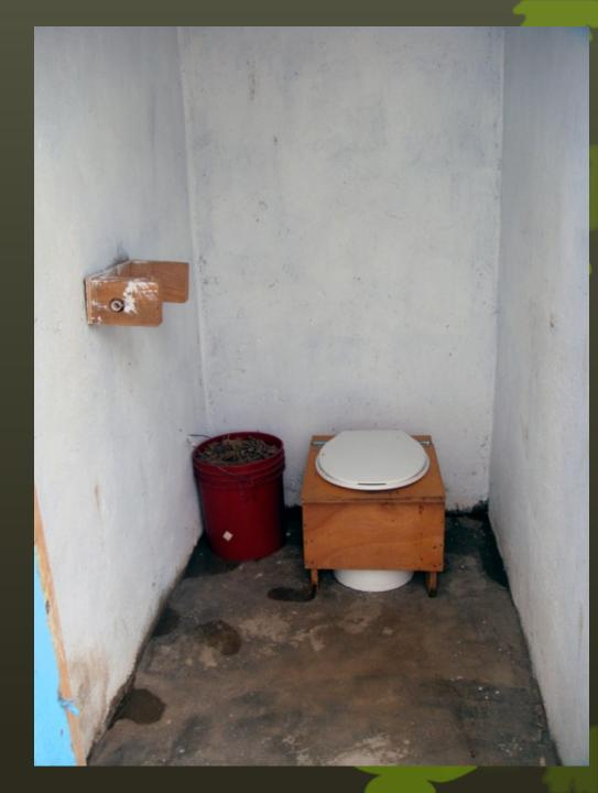
The contents are covered with the carbon-based material, which acts as a biofilter to prevent odor. The receptacle is easily removable.
